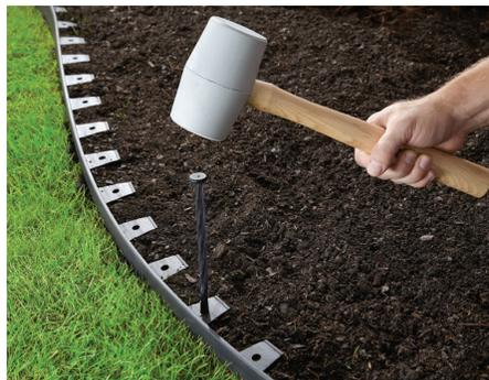
**2** Pound anchoring spikes through tabs to secure the edging. Typical installations require one spike every 2-3 feet.
