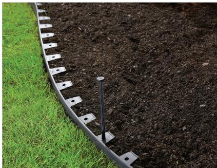
**1** Clear the installation area of loose soil and debris. Place edging on the cleared surface with anchoring tabs flat on the soil.
