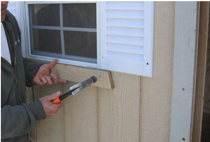
83. Next install the 2 3/4" bottom trim with 2" nails.
