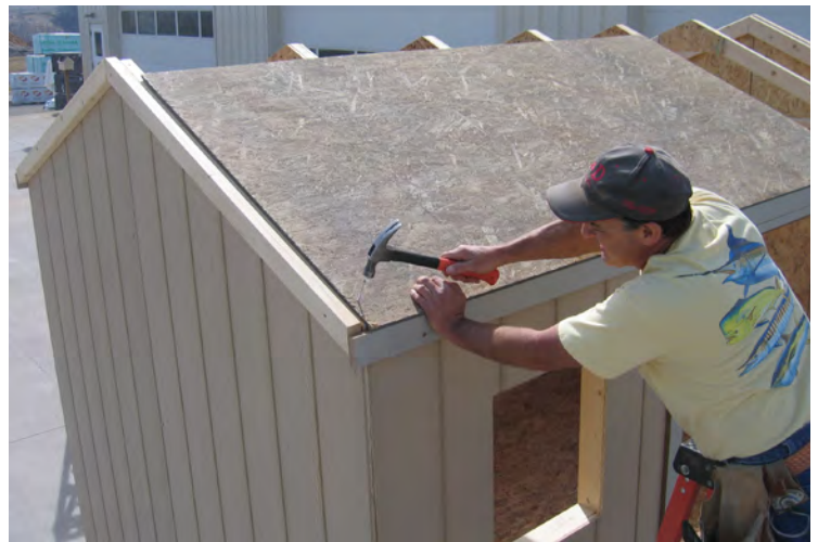
64. Next, following your ROOF LAYOUT sheet, install roof sheeting and fasten with 2" nails.
