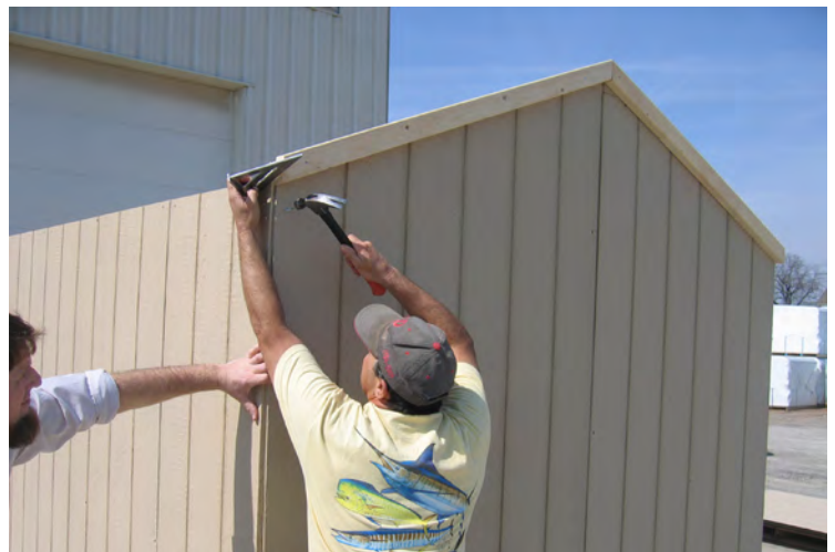
48. Fasten outside corner as shown with 2" nails.
