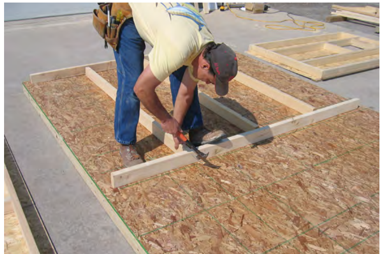
28. Secure with 3" nails as shown.
