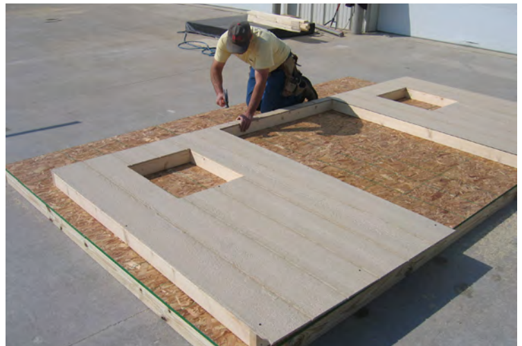
16. Fasten the header piece with 2" nails as shown.
