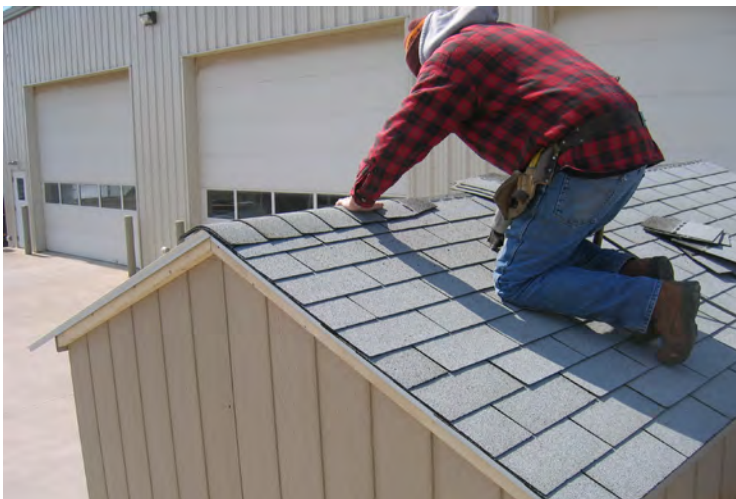
77. Continue placing the ridge cap, as shown.
