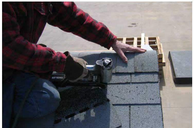
78. You can finish with a smaller cap with no adhesion strip.
