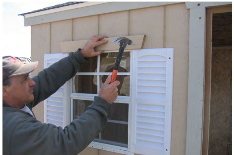
82. Install the top 2 3/4" trim piece as shown and secure with 2" nails.
