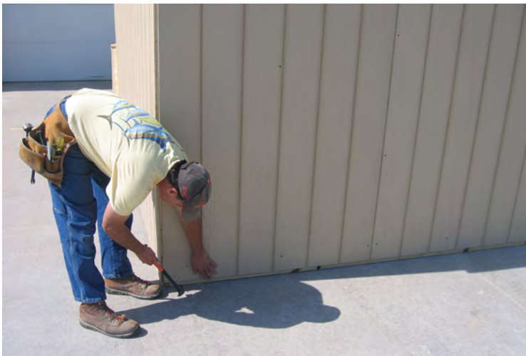
51. Next nail the bottom of the building with 2" nails 8" on center all the way around the building.
