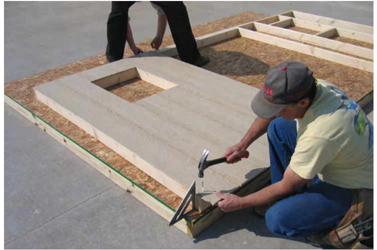
14. Make sure the outside corners are flush as shown before fastening with the 2" nails. Note: There will be a 3" skirt at the bottom.
