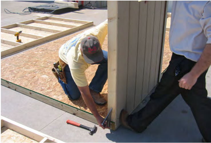
43. Make sure the wall is flush on the end and put pressure on the outside as shown, fasten with 3" nails.
