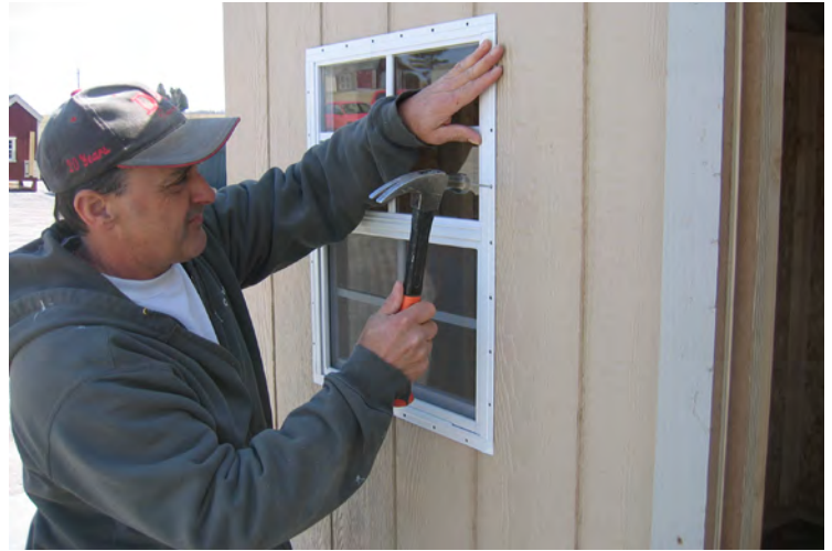
80. Install the window and fasten with 2" nails as shown.
