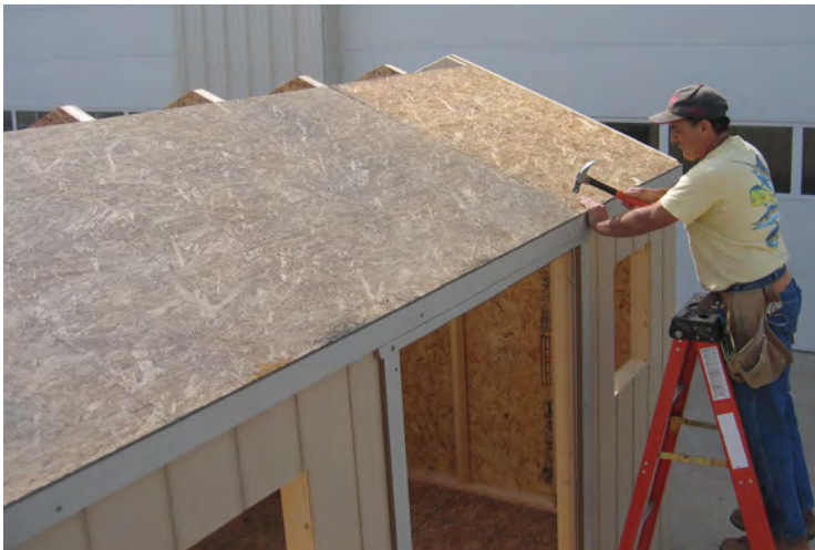
65. Continue with the roof sheeting.
