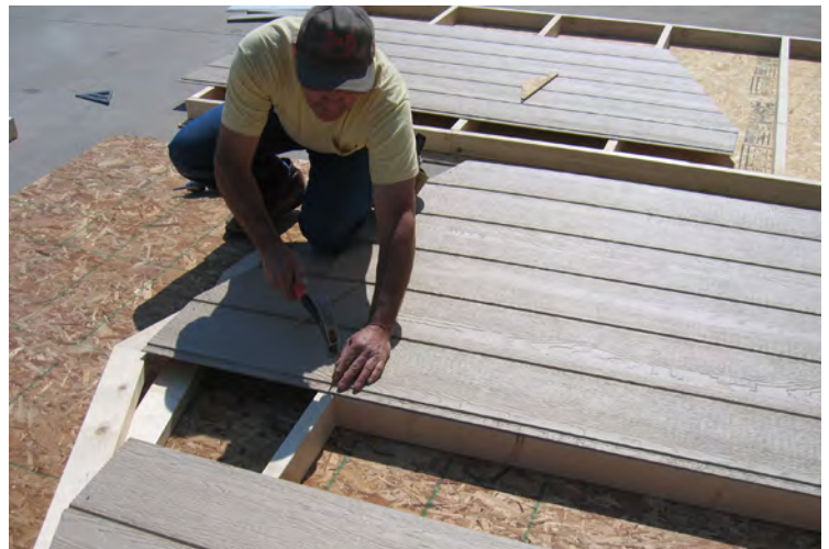
34. Secure with 2" nails every 6" to 8" on center.
