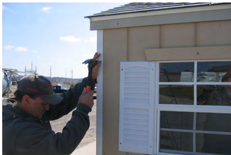
96. Locate the aluminum corner trim. Fasten the trim onto all four corners of the building with white finish nails.
