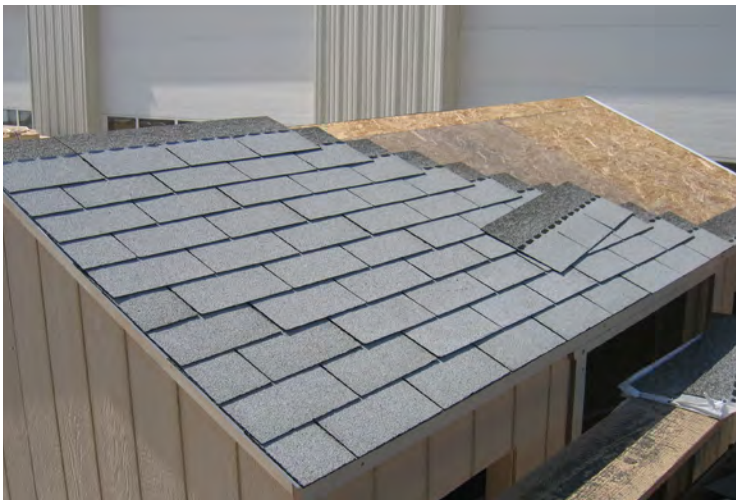
75. Continue with shingles as shown.
