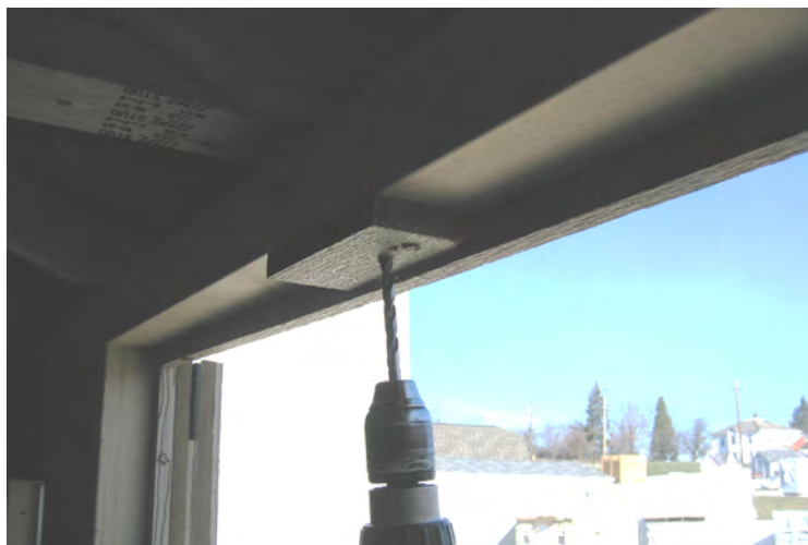
93. Drill a 5/16" hole for the barrel bolt.
