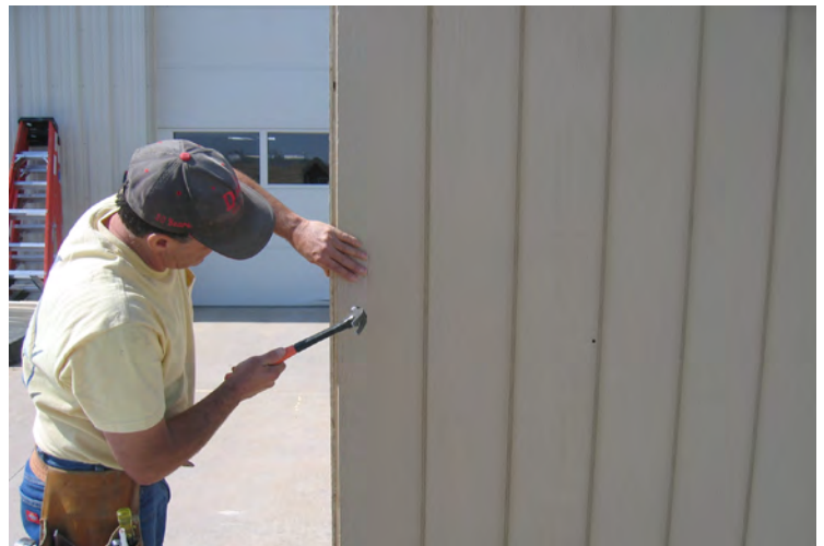
52. Nail the corners every 6" to 8" with 2" nails.
