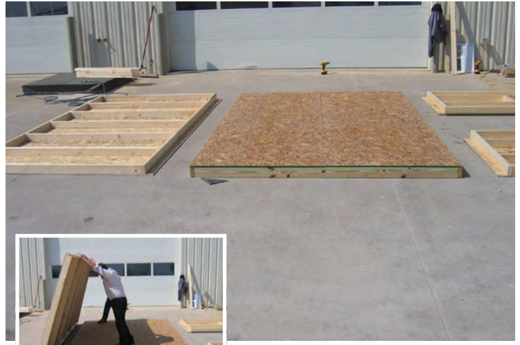
26. Lay wall to the side as shown.
