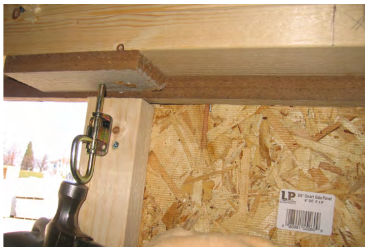
92. Tap on the top barrel bolt to locate where to drill your 5/16" hole.
