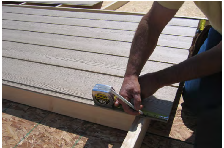
32. Refer to the SMARTSIDE LAYOUT SHEET for gable end siding placement. Install the Smartside making sure it is 3" from the bottom of the 2x4 to the bottom of the wall.
