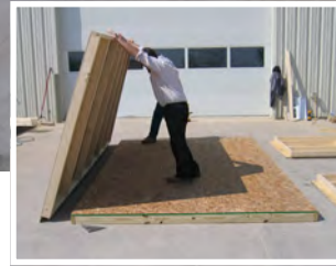
26. Lay wall to the side as shown.
