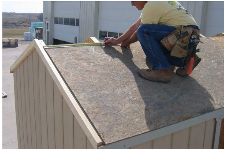
66. Make sure the trusses are 24" on center before fastening sheeting.
