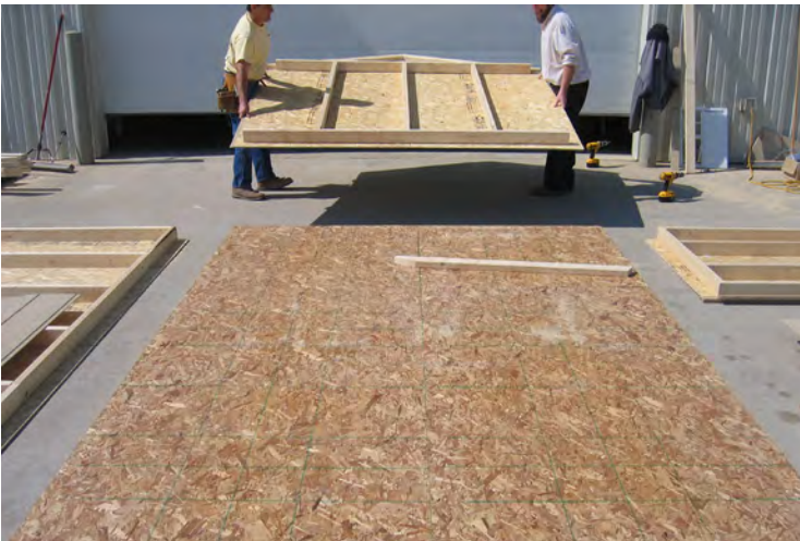
35. Lay wall to the side as shown.
