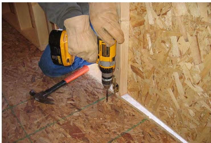
91. Drill a 5/16" hole as shown.
