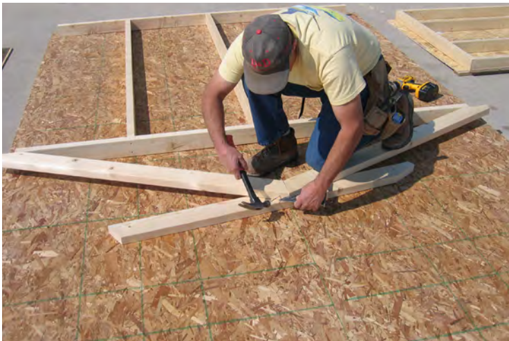
29. Using the WALL LAYOUT DIAGRAM sheet, locate the truss pieces, layout and fasten with 3" nails as shown.
