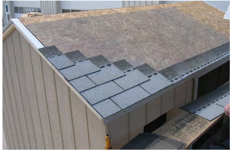
74. Install shingles in a staggered fashion.
