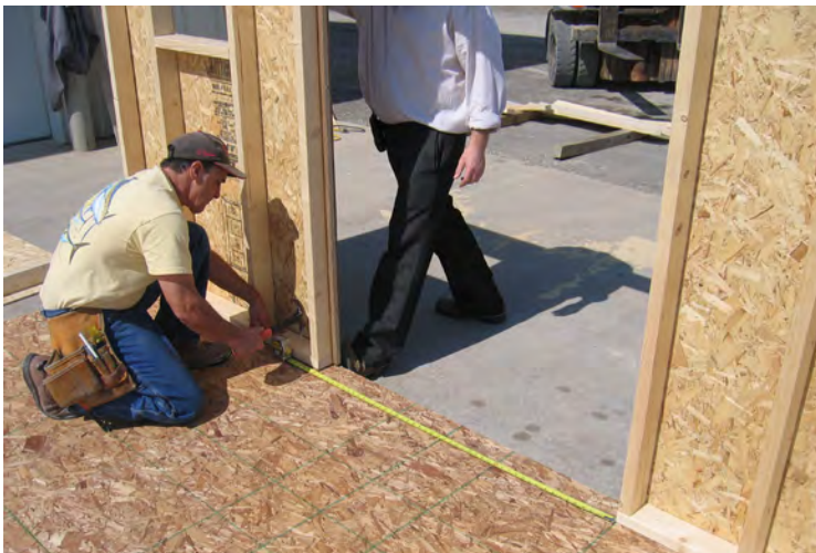
45. Make sure you have 48" or 60" (depending on the building width) in between the door opening, 48" on 8' wide buildings and 60" on 10' and wider buildings.
