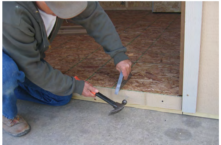
84. Locate 3" Smartside siding pieces and keep flush with the top of the floor and secure with 2" nails.
