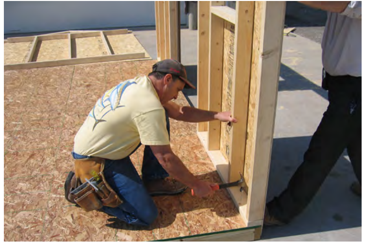
44. Fasten with 3" nails 16" on center.
