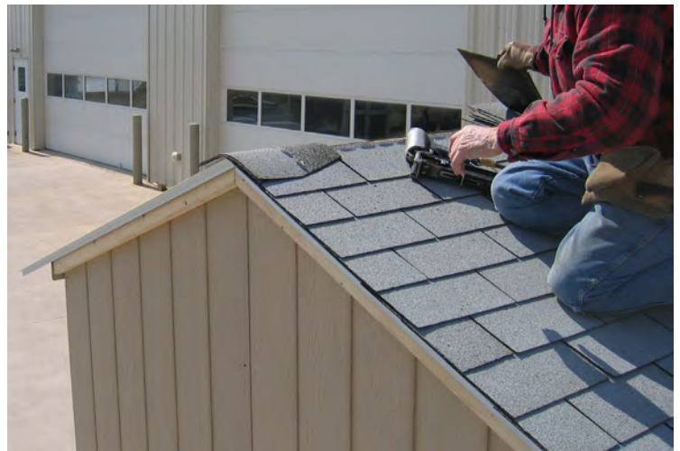
76. Cut the ridge caps and install the first one as shown.
