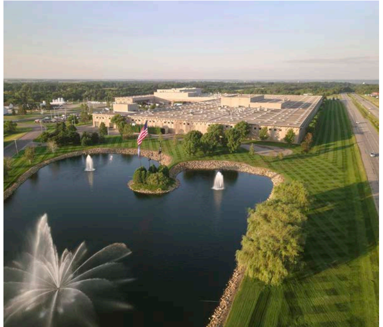
CAMBRIA SLAB MANUFACTURING FACILITY Le Sueur, Minnesota
