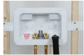
Right drain, box mounted center
