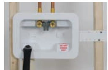
Left drain, box mounted on left stud with valve on top
