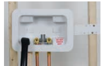
Left drain, box mounted on left stud
