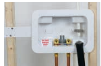
Right drain, box mounted on right stud with secondary drain line
