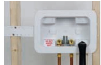
Right drain, box mounted on right stud
