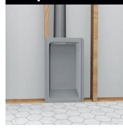
Attach the Dryerbox to a wall stud and bottom plate. A minimum of 3 corners is required.
