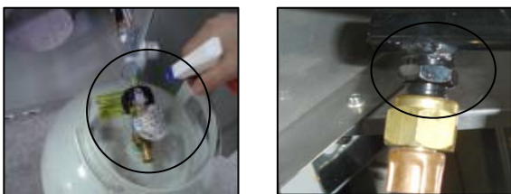
Gas Connection Leak Check
