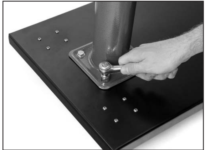
Figure 6. Installing collector support.
