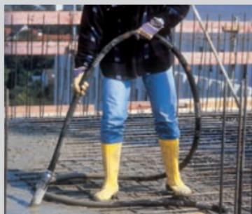
These high-frequency motor-in-head vibrators feature a unique integrated converter that allows the units to plug directly into a standard 115V outlet. This patented system gives you the performance of high-frequency without an expensive high-cycle generator. The micro-inverter automatically changes single phase 60 cycle to three phase 200 Hertz which guarantees consistent RPM with no loss under load.
