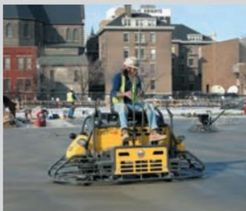
These 48-inch ride-on trowels offer high productivity and quality results. Featuring a patented torsion assist steering system, these trowels are easy to operate and reduce operator fatigue. Ergonomic twin lever control makes for excellent maneuverability.
