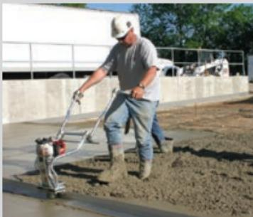
A wet screed that can fit the demands of every job site with a variety of blade lengths, plus each unit is designed to fit the demands of every operator. Its unique twin handle system is fully height and angle adjustable offering maximum operator comfort.
