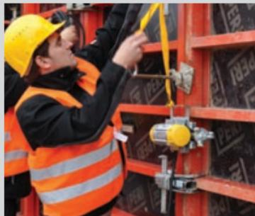
The AR 26 external vibrator was designed specifically for cast-in-place formwork as well as light precast concrete applications. Its low weight, compact size, and ability to keep a constant speed under load make it the preferred external vibrator for concrete consolidation. Accessory clamping devices are available and are designed to be lightweight, portable, and efficient.
