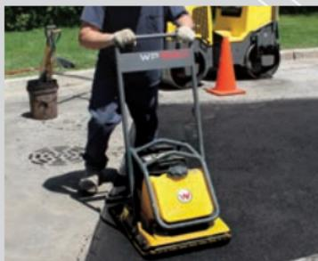
Designed for the compaction of asphalt as well as granular and mixed materials with some cohesive content in confined areas. Large capacity, semi-transparent polyethylene water tank with filter, located within the front lift cage for protection.
