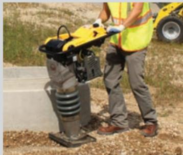
The preferred vibratory rammer design in the industry is available with a WM 100 or a Honda GX100 4-cycle engines. These Rammers are designed for the compaction of cohesive, mixed and granular soils in confined areas. Exclusive air filter compensation system for longer run time between filter changes.
