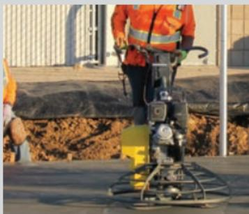
These variable speed trowels will get the job done... fast. A variable transmission system provides wide speed range (25-200 rpm) for low-speed, high torque floating through high-speed burnishing all in one machine. The large pitch-control range offers complete control over finishing and floating for application versatility during operation.
