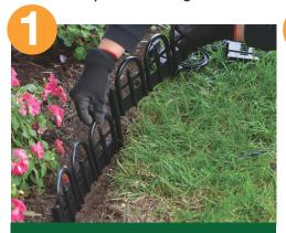
Clear the installation area of grass, loose soil, and debris. Slide edging pieces together so anchoring tabs overlap.
