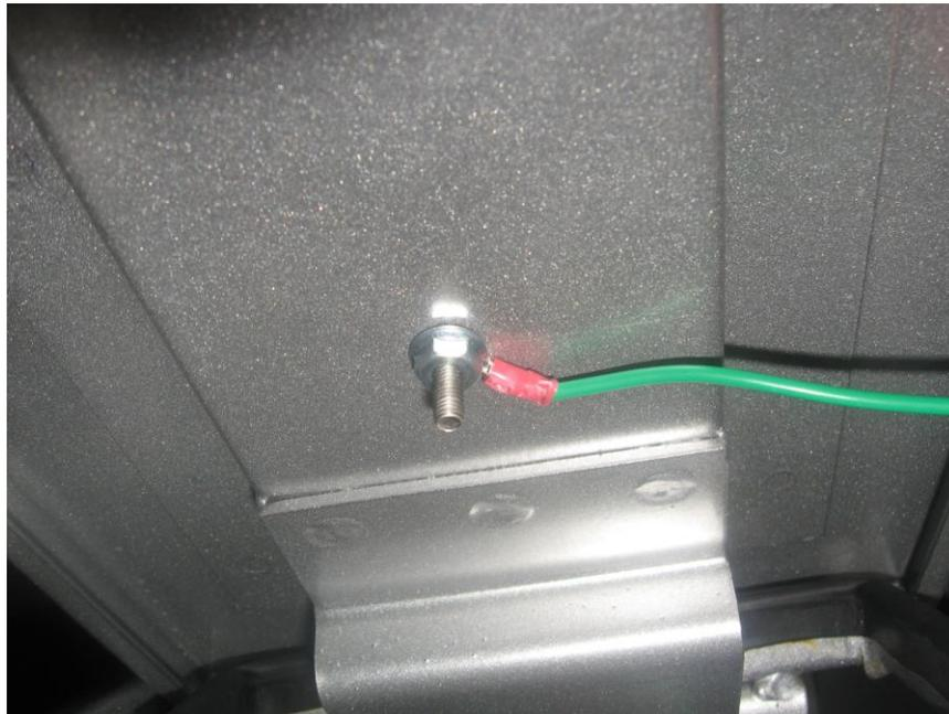
Figure 49: Door Ground Connection
