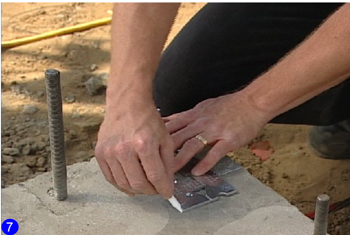
7 Complete the second mark by marking along the tool's ruler edge.
