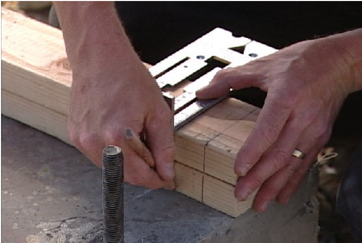
Stack top and sole plates
