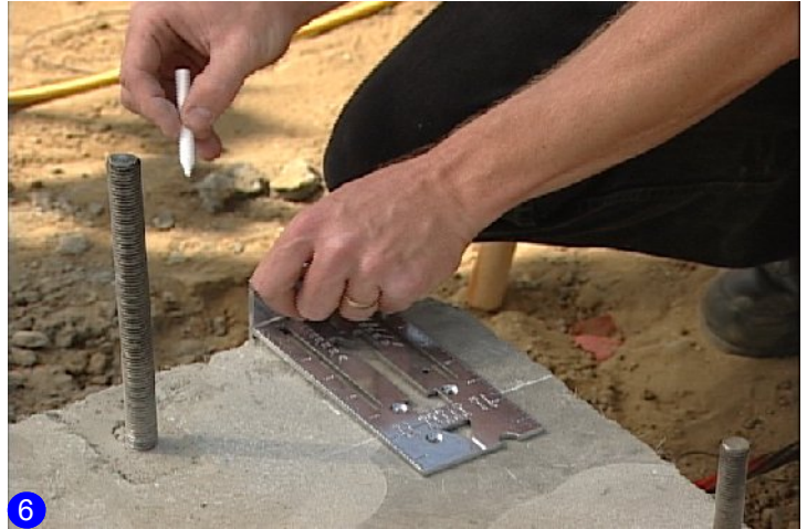
6 Line up tool with previous mark.
