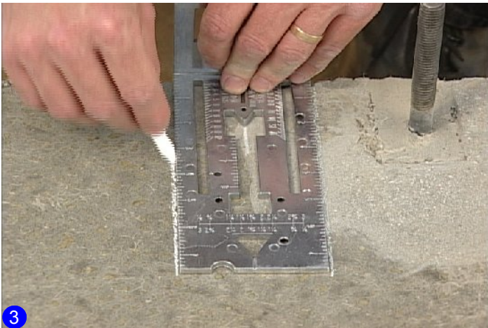
3 Make marks on both sides of tool.
