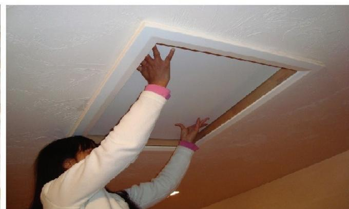
**3. Fasten frame into joists or trusses.**
