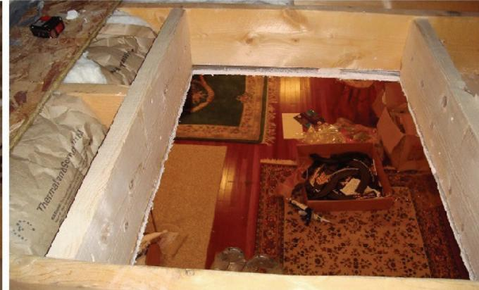
**1. Select location. Door fits between trusses 24" o.c. or between joists 16" o.c. Rough opening 22 1/2" x 30 1/2".**
