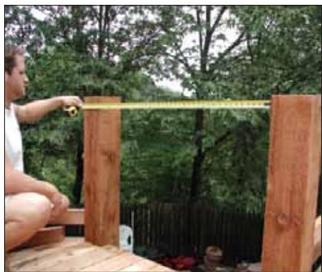
**Step 1:** Measure railing opening, from post to post.
