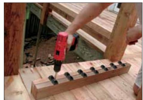
**Step 3:** Screw on connectors on each mark.
