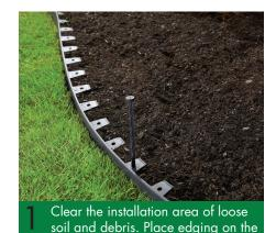
cleared surface with anchoring tabs
