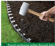
Pound anchoring spikes through tabs to secure the edging. Typical installations require one spike every
