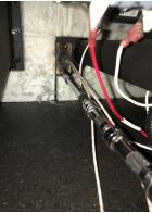
6. Use a 1/8" allen wrench to loosen the set screw while holding the igniter in place in the igniter housing.
