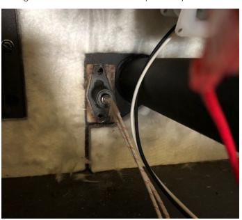
11. Reconnect the two wiring leads back into the wiring harness.
