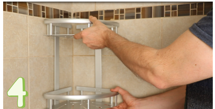
4 Put shelf on the wall and Do not tighten the sticker screws
