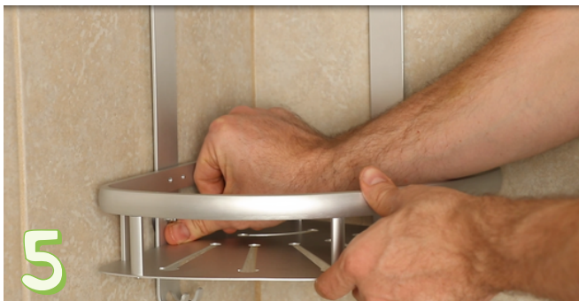
5 Squeeze out the air for the sticker and Tighten the screws after 24 hours
