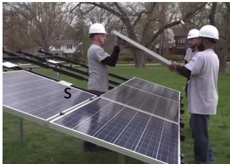
and place panels as required securing the bottom panels first.
