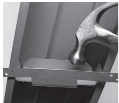
FIGURE 13 DRYWALL STUD ANCHOR INSTALLATION ON FRAME
