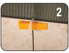
Slide the reusable wedges into the clips to level, align, space and hold the tiles.
