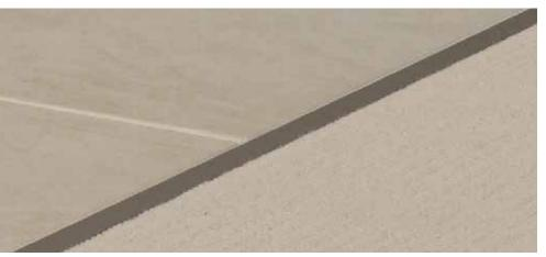
RENO-TK floor profile used to create a smooth transition between the tile and carpet. RONDEC bullnose profile and matching corners used to finish the edges of the tile base. DILEX-EKE PVC corner movement joint profile used to create a seamless transition between the floor and wall.
