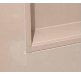
QUADEC square-shaped profile and corners used to finish the tile edges on the wall, shower curb and niche. DILEX-EKE PVC corner movement joint profile used to create a seamless transition between the shower walls and floor.
