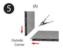
For outside corners (A) or inside corners (B), mitre cut both adjoining sections. Notch the front edge of one section to create an overlap.
