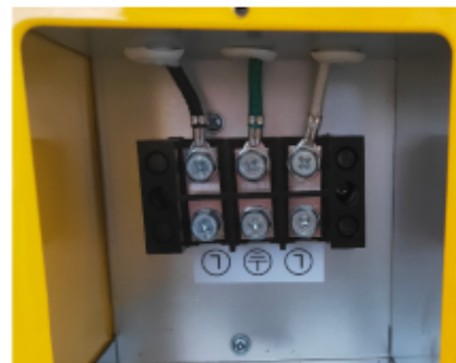
Figure 10 Removing wiring cover exposes wires When wiring with 2 conductor cable with ground, the white wire must be marked black.
