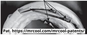
If the screw connections are tightened with too little torque, they will leak. If they are tightened with too much torque, the screw connections could suffer damage. Please refer to the torque requirements section for more information. If you do not feel confident connecting the line set connectors yourself, it is imperative that you contact the MRCOOL® customer service team or an HVAC professional.
