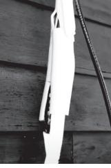
3. Now, starting where the line set is not covered with the factory plastic (close to the indoor air handler connection, you will wrap the line set upward to the wall hole, using the supplied Non-adhesive U.V. tape. This will cover the insulated line set connections, cables, and drain hose. The drain pipe will need to be at the bottom of the bundle (**Refer to Fig. 7.2**).
