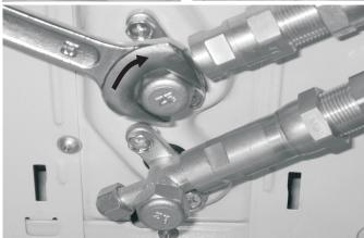
2. Using the images below as a guide, repeat the same process for the bottom valve. Remove the cover on the bottom valve, using a 19 mm open-ended wrench or a crescent (adjustable-type) wrench. Then, insert a 5 mm Allen key and open the valve by turning it counter-clockwise as far as it will go. **DO NOT** force it. Screw the cover back onto the bottom valve and tighten it well to ensure that it is properly sealed.
