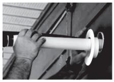
2. Place your hand on the underside of the piping coming through the exterior wall hole (from indoor unit), close to the wall. With your other hand, using even pressure, carefully bend the piping downward toward the wall, being mindful not to damage or dent the piping in the process.
