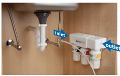
8. Connect the supply lines: push the tubing into the inlet side and outlet side of the housing. The tee fitting tube goes to the inlet and the faucet tube goes to the outlet.
