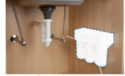
4. Unit installation: Select a space under your sink for the filter unit that is at least 12 inches from the bottom of your cabinet and allows for easy access to your cold water supply and for filter replacements. Use a pencil to mark wall screw placements.
