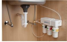
9. Turn the cold water on. Check for leaks and proper installation: place a towel under the filter unit and check for leaks. Allow water to run for 10 minutes to flush carbon fines. Note: Never use oils to lubricate the O-rings; O-rings come pre-lubricated.
