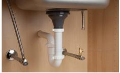
2. Brass Tee Installation: Attach threaded ends of supplied brass tee to the cold water supply line and shut-off valve; tighten using an adjustable wrench.
