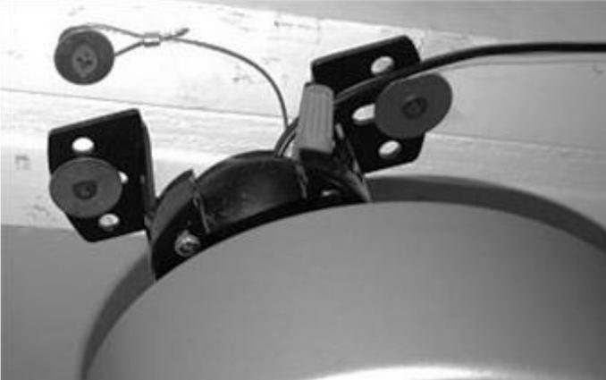
**Photo 5:** Safety cable attached near hanger
