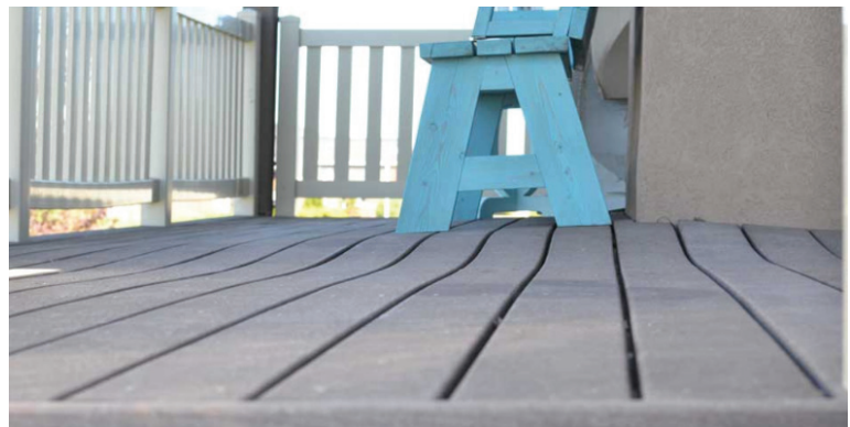
Example above showing the effect on decking when attached to uneven joists/framing.
