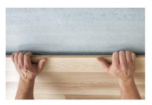
Connect the planks in the following rows by repeating the process of applying adhesive to the back of the planks, engaging the length side tongue and groove, along with the short ends, and fastening the engineered hardwood with a brad nailer through the tongue in the wall stud.
