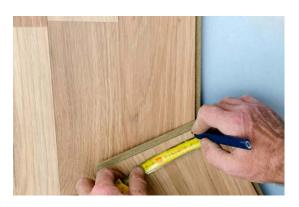
The last row of the laminate may need to be cut. Measure the distance between the finishing walls To the last row of engineered hardwood that was installed and using a table saw or jig saw cut the laminate to the width desired.
