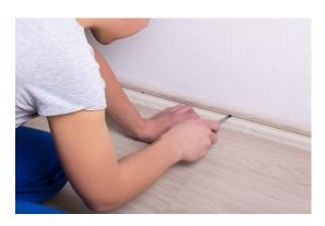
Remove existing baseboards on the wall that will be receiving the engineered hardwood.
