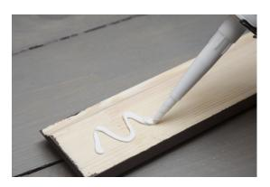
Using a construction adhesive put an s-bead of adhesive on the back of the planks.
