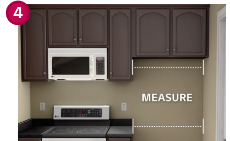
Measure the width of the opening at the countertop, under the upper cabinets and at the base if there is a molding.
