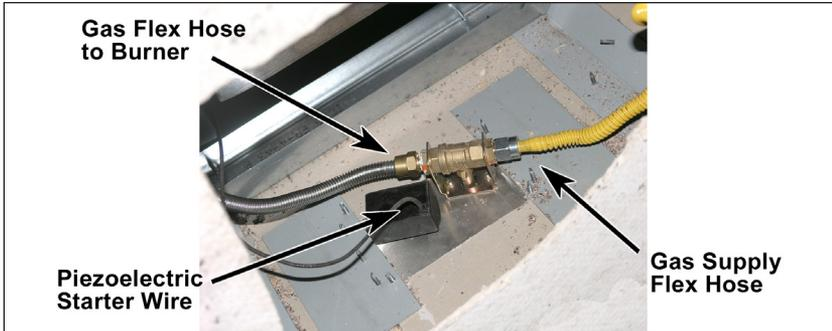
Place the fire pit back down on its pedestal. Attach the gas flex hose to the burner.
