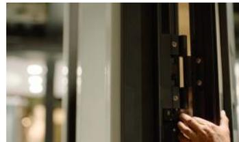
Step 6: Set the hinge pin when the hinges are aligned and tighten the hinge pin security screw with the T-10 bit. Place the hinge caps at the top and bottom of each hinge.
