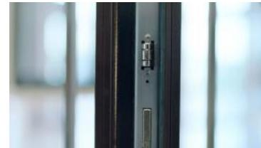
Step 9: The hinges allow for horizontal and vertical adjustments to the door. To make adjustments, loosen the two large screws using a T-25 drill bit. This allows the hinges to freely and safely move in the next step.
