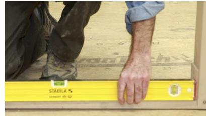
Step 3: Anchor the frame with #12 x 3 in. screws using the pre-drilled installation holes at the top and bottom corners. Be careful not to over tighten or strip the screws, and recheck for plumb, level, and square when finished. Shim and anchor the frame through the remaining pre-drilled installation holes, taking care not to bow the frames when shimming.
