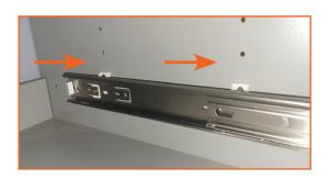
In a standard base cabinet there is a location on the inside for the roll-out tray. Indicated by the two sets of pre-drilled holes on the back panel.
