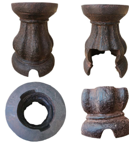
C. Top pedestal and pump access door
