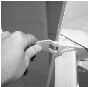
Tilt Latch Figure F
