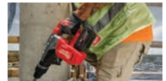
Drilling multiple back-to-back holes in concrete
