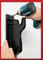
2. Attach straight up and down to the stud.
