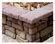
**Step 4**: Install the caps. Start at a corner and place a cap on the planter leaving approximately a 1" overhang. Continue placing caps around the planter making slight adjustments as needed to get the caps in place. Cap overhang may vary. You will need 10 caps for the square planter and 15 caps for the rectangular planter. Remove the caps one at a time and adhere each cap to the blocks below with a quality concrete adhesive.
