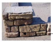
**Step 3**: Install second course of blocks. Place a corner block on top of the bottom corner block staggering the intersection of two blocks on the course below. Continue around the planter making slight adjustments as needed so that the edge of the blocks fit tightly. Remove the blocks one at a time and adhere each block to the blocks below with a quality concrete adhesive.
