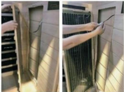
3 Disconnect the connection line between the heater and the sauna wall;
