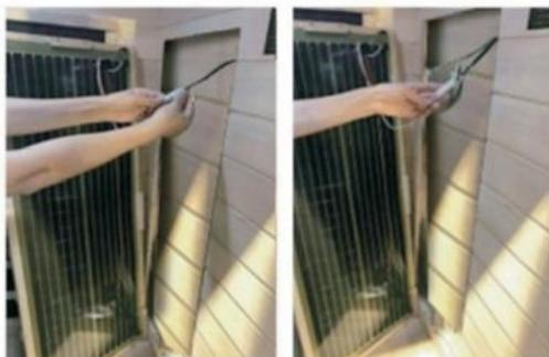
6 Fix the replaced heater and grate on the sauna wall.
