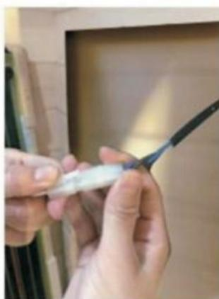
4 Remove the heater to be replaced from the wooden fence and replace it with a new heater;
