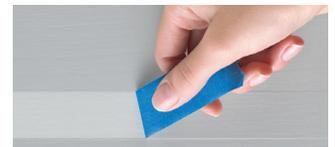
Remove tape at a 45° angle. If adhesive begins to transfer, use a 90° angle. If paint starts to lift, use a sharp tool to cut along the painted tape edge.
