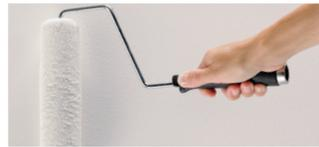
Paint the basecoat (the lighter color) over the entire wall and let it dry for 24 hours.
