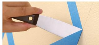
Tape the outside edge of every other diamond. Press down to seal all edges of the tape.
