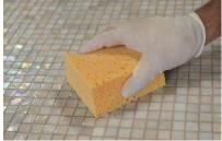
If the white pad / felt and soft sponge becomes impregnated with resin and can no longer be cleaned, they should be replaced.
