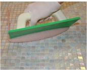
The standard and optimum temperature condition for application is between 65 and 75°F. Under these conditions, the product appears like a soft, easily workable paste, with a workability time of approximately 1 hour.
