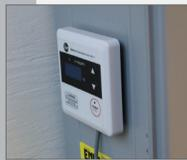
With no fixtures running, turn on the water, the gas, and the electricity to the water heater. Wait 90 seconds to allow water heater to complete start up system checks. Press the Power button on the remote control as it will beep and a green light will come on. The remote will display "100" the first time you turn it on.
