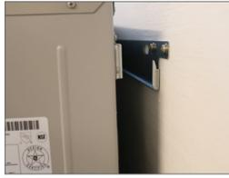
the bottom. Use washers to ensure the water heater is secured.
