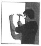
Wait for adhesive to set up, but still be tacky Apply panel to wall, position as needed, press into place Use paneling nails to secure panels, along with adhesive
