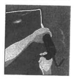
Use quality construction adhesive (i.e. Loctite PowerGrab) Extrude a bead 1/4" in diameter, or less, around the perimeter of the panel and vertical lines 12" or 16" O.C.
