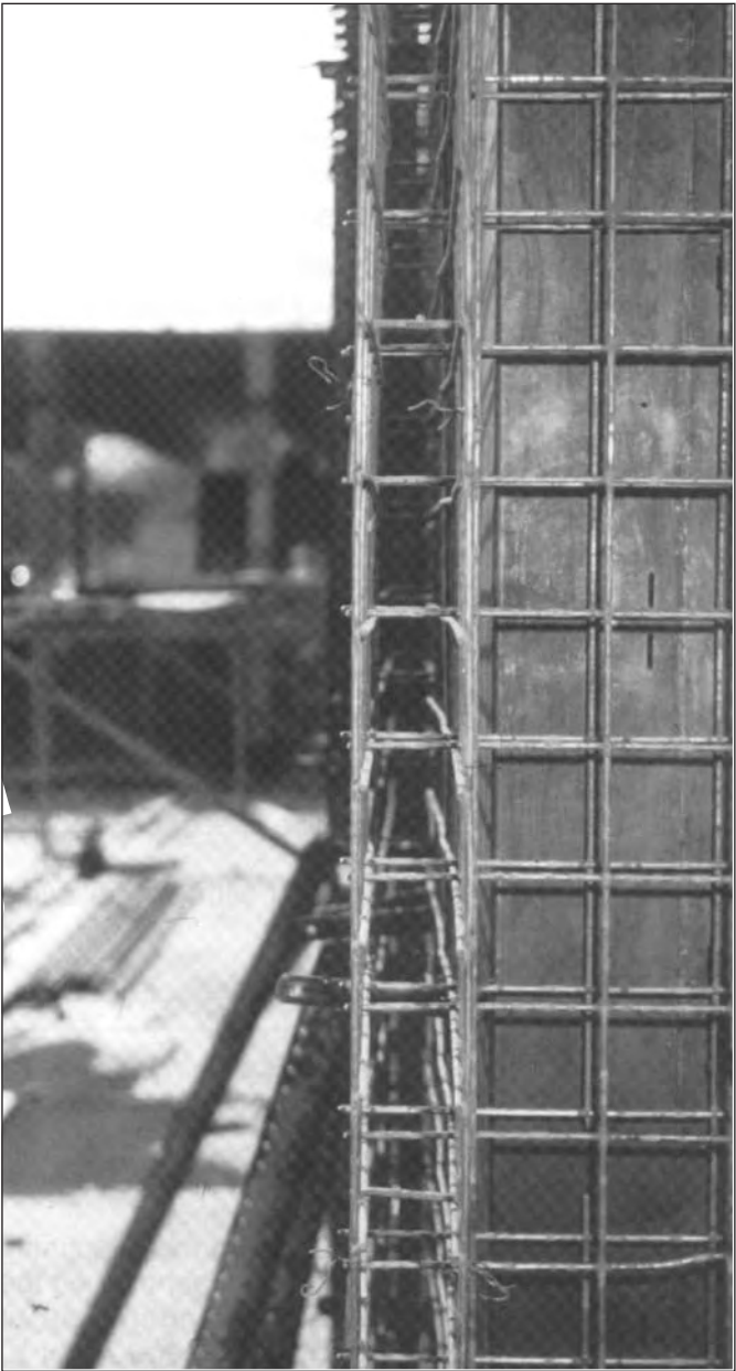
(Above) Inner and outer vertical face of wall reinforcement.
