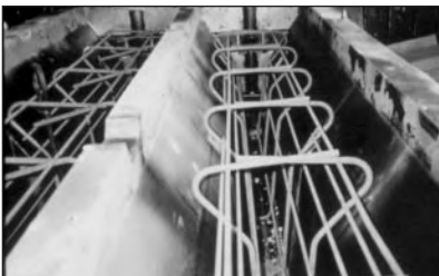
WWR used in highway median barriers.
