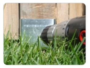
**Step 5:** Preferred method, fasten with a #8x1.5inch self-tapping stainless steel screw. For **Vinyl installation** pre-drill a hole then fasten with same screw with mild pressure so as not to deform Armor.
