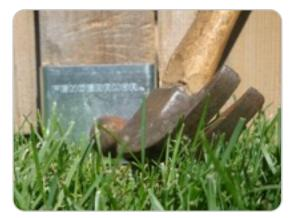
**Step 4:** If desired, use a hot dipped galvanized nail, 1 inch to 1 1/4 inch long. Hammer into place.
