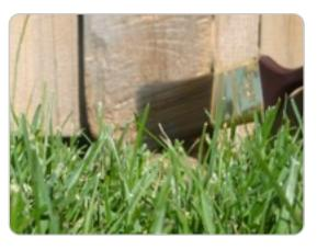
Step 2: If your post is already damaged, it is best to waterproof, stain or paint the effected area before installing Fence Armor.
