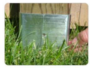
**Step 6:** Fence Armor can also be fastened from the sides, aligning hole to slot, if accessible. This is optional, in most cases this is not necessary.
