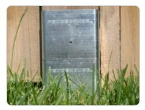
**Step 7:** If a larger vertical area of protection is required, Fence Armor can be stacked until desired height is attained.
