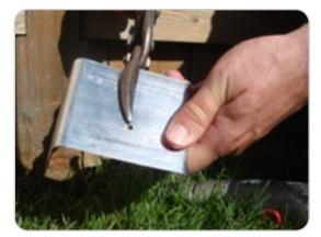
**Step 11:** Cut Fence Armor down the centre to achieve a 90 degree corner. Again, do not forget to round the corners.
