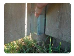
Step 12: To fasten, pre-drill a 1/8inch hole in an accessible location, & fasten as described in steps 4 or 5.
