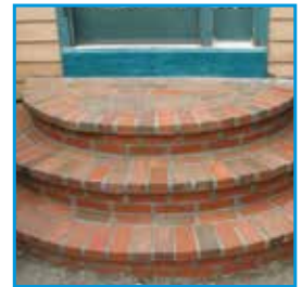
Repair Chipped Brick
