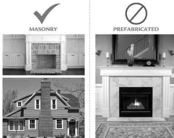
A. Masonry Fireplaces are constructed of brick and mortar with a brick chimney.
