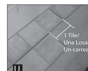
For repeating uniform size face pattern flooring: TO CREATE A UNIFORM BLOCKED DESIGN, stagger the end joint (where planks meet) of the plank being installed a minimum of one tile on the face pattern design. This will ensure that the planks being installed "row. Align the tiles face joint/grout pattern END JOINTS IN ADJOINING ROWS SHOULD BE STAGGERED 12".
