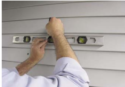
DRILL (4) 1/2" CORNER HOLES THROUGH WALL FROM INTERIOR AND CONNECT HOLES ON EXTERIOR WITH A LEVEL.
