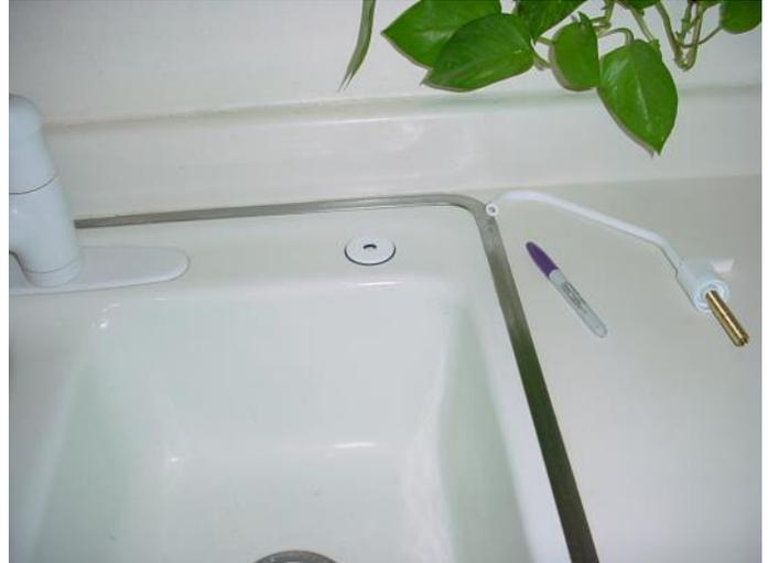
conditions are met. Mark center of base cover plate with marker. Place towel underneath sink, below drilling site, to collect fillings. Always wear protective eyewear and gear while drilling, and while under sink.
