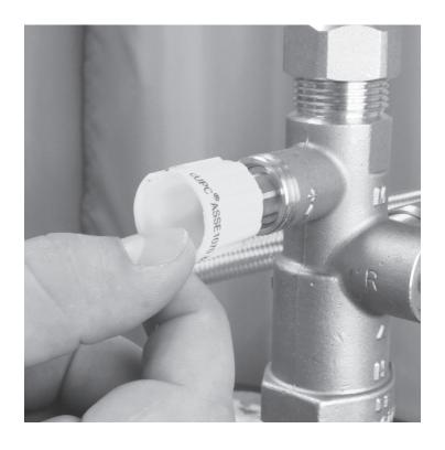
4. Turn cap 1/4 turn counter-clockwise (to the left) to increase water temperature to your house by 5° F. Turn cap clockwise (to the right) to decrease water temperature.
