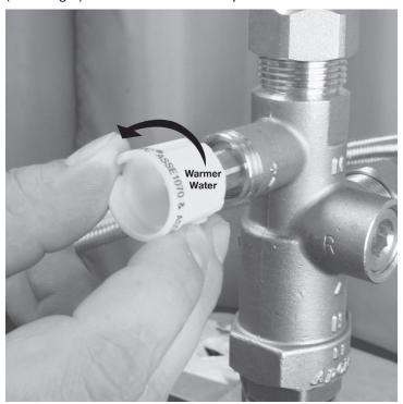
If your water heater is set to 140° or above, the mixing valve is factory pre-set to produce hot water at 120° F. The lowest setting for the valve is 100° F. The highest setting is the temperature at which your water heater is set.
