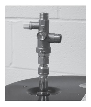
3. Connect the tee to the cold water inlet of the water heater.
