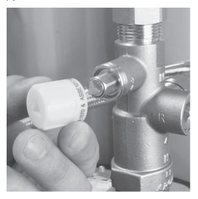
3. Place cap triangle end on the brass triangle on the mixing valve.
