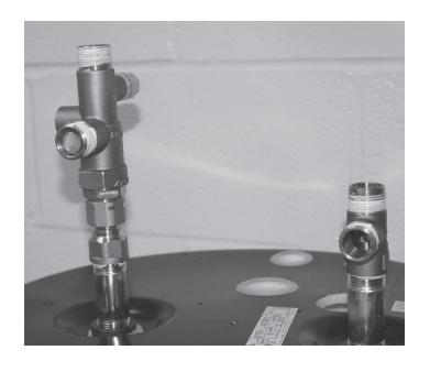
5. Connect the flexible hose from the mixing valve to the tee as shown below.
