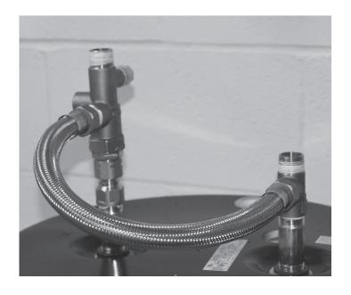
6. Connect the system's cold water inlet supply hose to the tee and the hot water outlet supply hose to the mixing valve. Turn on water and check for leaks.
