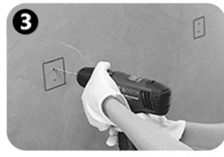
Drill screw mounting holes on thewall.
