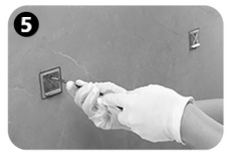
Fix the gasket of the product on the wall with phillips screwdriver.
