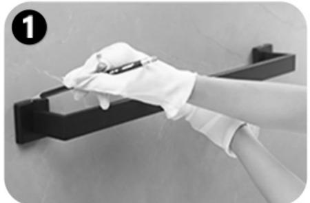
Determine the desired height and position and mark it.
