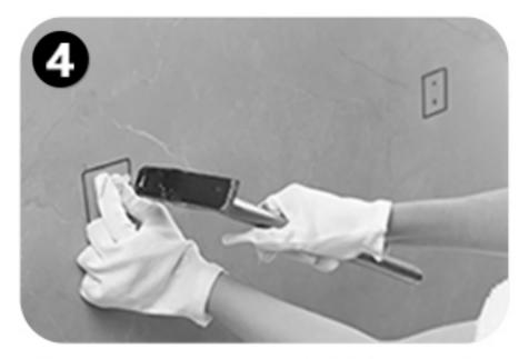
Using a hammer to hit the anchor into the holes.
