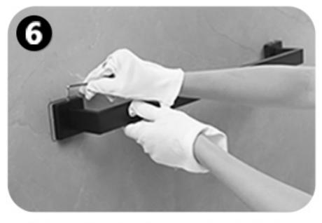
Using the "L" tool to install the other parts of the products.
